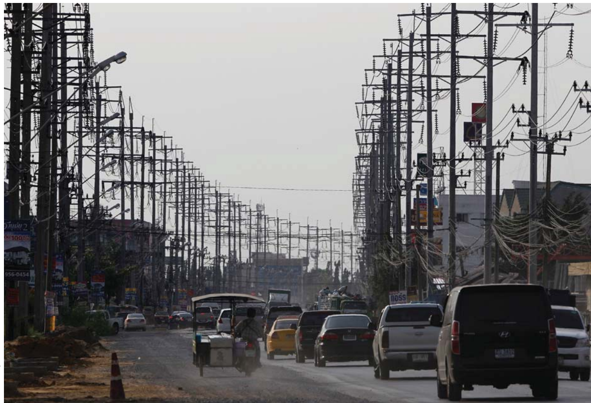
Vehicles drive along a road near electricity posts in Thailand's Nonthaburi province.
