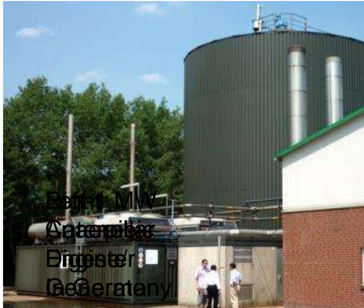
Left-1 MW Anaerobic Digester In Germany
