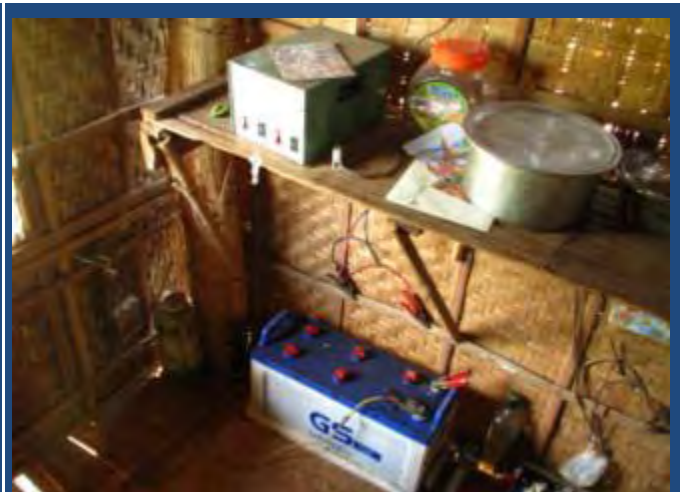
Badly protected battery of a makeshift SHS - provided for free and without user training
