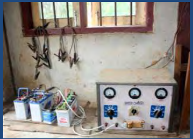
Pico hydro powered business: battery charging to run TV and DVD
