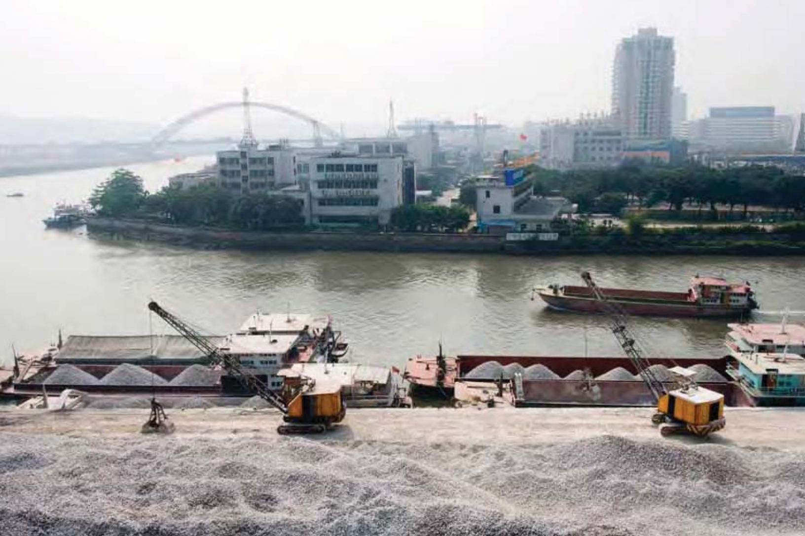
Factory beside the river: Water is a critical input for industry, agriculture, energy production, and the tourism and service sectors.
