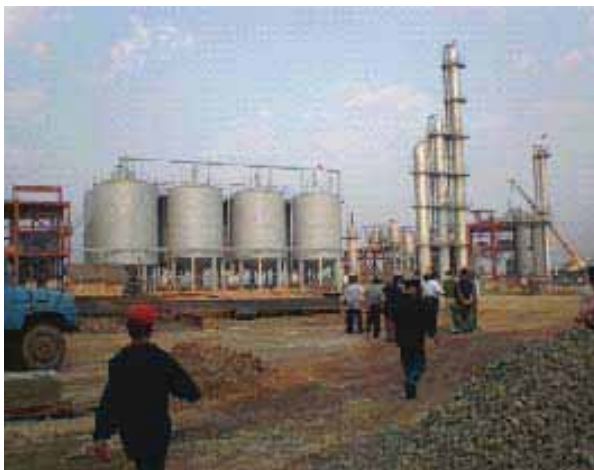
Figure 37: Ethanol Plant Under Construction at Maunggone Village, Tagaung Township, Sagaing Division
