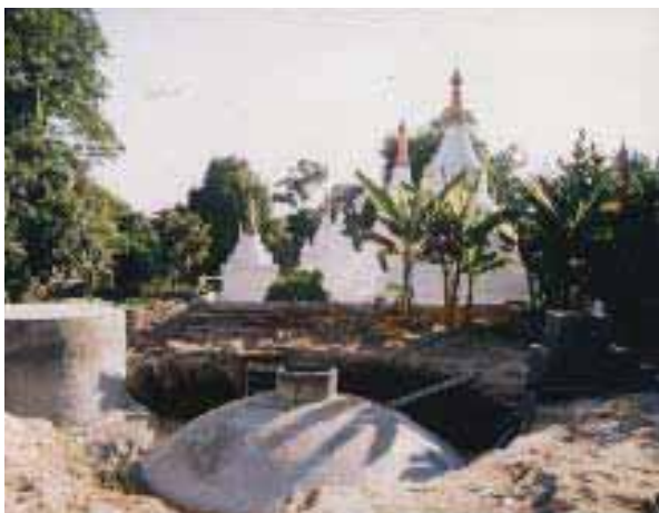
Figure 20: An Almost Completed Biogas Unit
