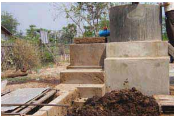
Figure 15: Fixed Dome-Type Biogas Plant
