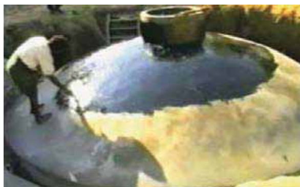
Figure 19: Fixed Dome-Type Biogas Tank (50 m 3 ) Under Construction
