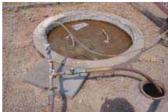
Figure 15: Fixed Dome-Type Biogas Plant
