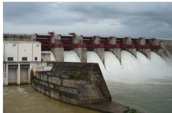
Sedawgyi Hydropower Station
