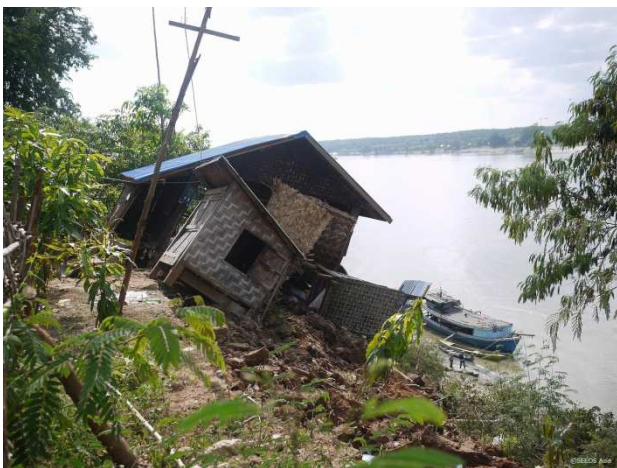
Houses on river side has been tilted due to landslide after the earthquake.
