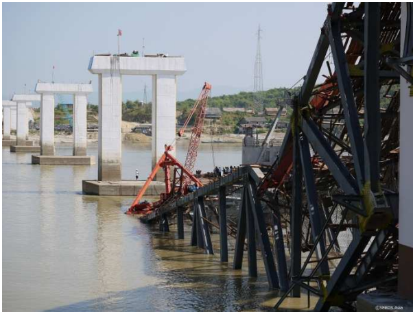
Yadana Theinga bridge in Kyaunk Myaung Township in Shwebo District, Sagain Region photo taken from the construction project office of Public Works, Ministry of Construction. The bridge with the weight of 910 tons was being under construction and failed into the river by the earthquake. One worker was killed. 18 workers were injured as of 13 th Nov.2012
