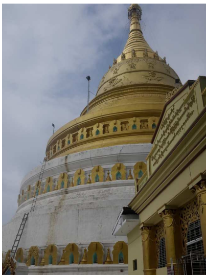
15 damages were found. [Htu Par Yone Pagoda]
