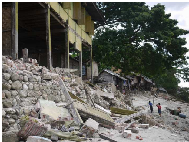
Houses along the river are damaged and people evacuated and remained outside.
