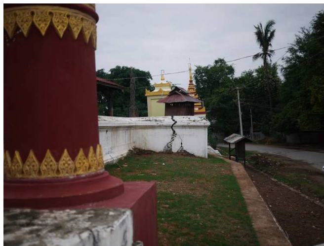
Damaged piece from Pagoda. Very light and soft materials were used for the building [Maha Myngalar Pagoda]
