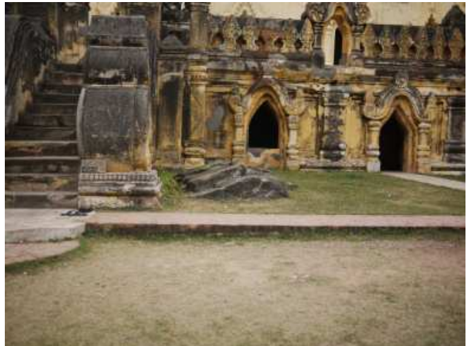
The stone on the right side of the entrance shows the sign of the existence of fault. [Maha Aungmyay Bonsan Manastery(Manu building)]
