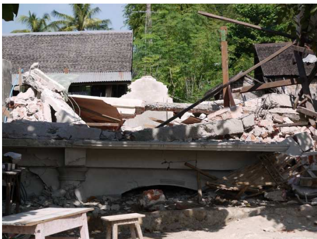
A house totally collapsed in Thabeikkyin township. It has been nine months since it was built.
