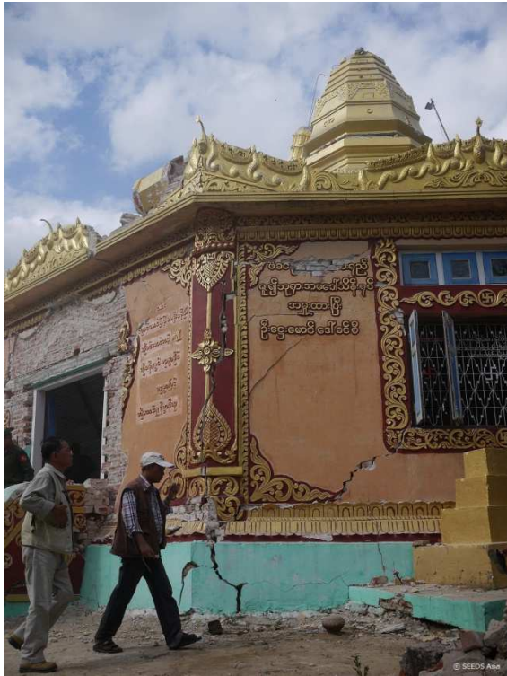
Damaged Pagoda and walls.
