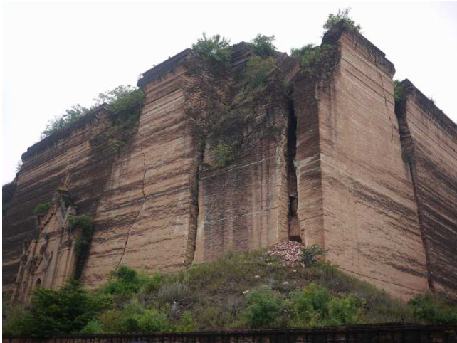
New cracks came out and the existed cracks on the building got wider than before due to the earthquake.
