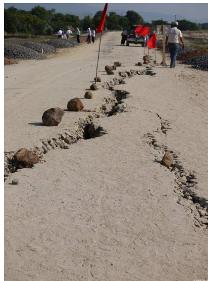
Ruptures on the approach way to the Yadana Theinga bridge, Singu Township
