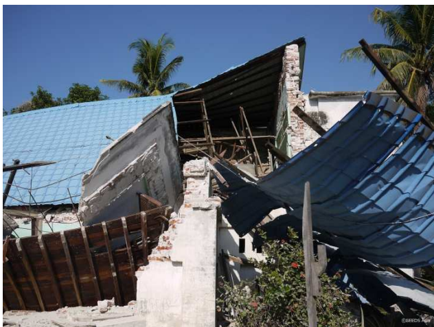
A building in Basic Education Post Primary School compound, Khule village, Singu Township
