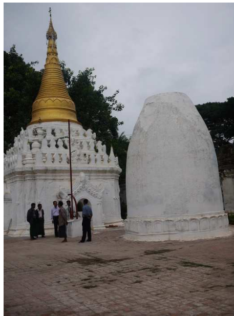
Previous earthquake hit this pagoda, and the top side of the pagoda was dropped and set in the compound. [Lawkatharaphu Pagoda]
