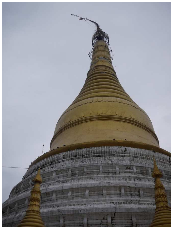
Pagoda was damaged [Maha Mingalar Pagoda]
