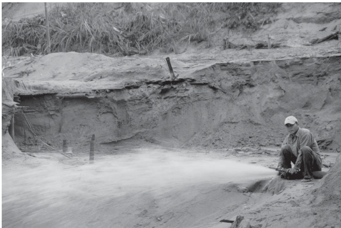
Photo 14: Water blasting of the riverbank.
