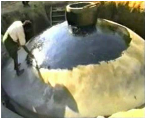
Fixed dome type biogas tank (50 m 3 ) being constructed. (Courtesy: MES)
