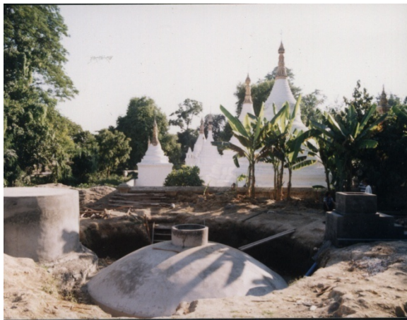
Almost completed biogas unit.
