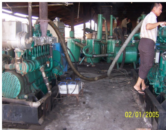
Wood chip gasifiers and generators in JLC, Mandalay.
