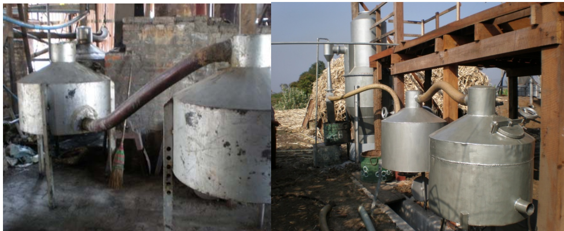
Small scale rice husk gasifier in a "Pwat Yay" factory, Tagaung. Gasifier at "Mann Myo Daw" Sugar Factory, Mandalay.
